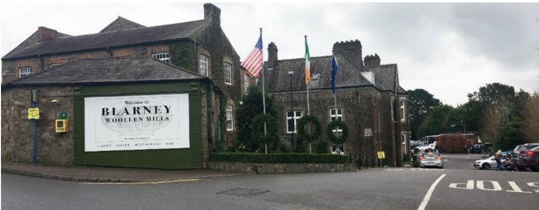
Photograph 10 Protected Structure, Blarney Woollen Mills
